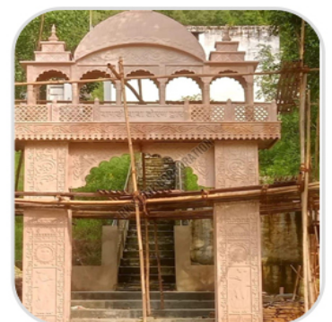
Heavy Duty Sandstone Entry Gate for Temple
