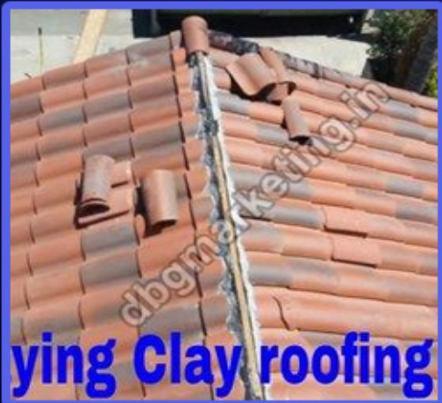
Laying Designer Clay Roofing Tile
