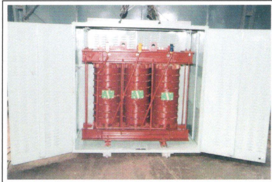
Dry Type Transformer (400 KVA)
