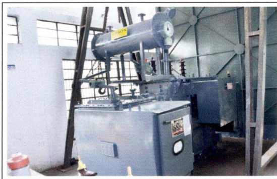
Power Transformer 33/433 KV, 1000 KVA
