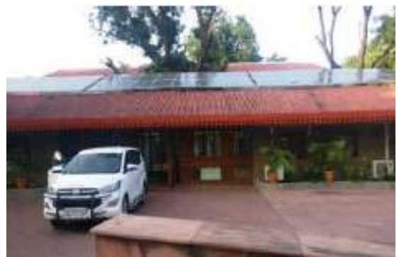
30 KW GOVERNOR HOUSE, GANDHINAGAR
