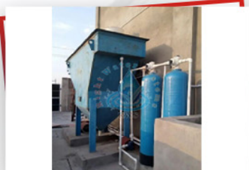
10 KLD Prefabricated Effluent Treatment Plant
