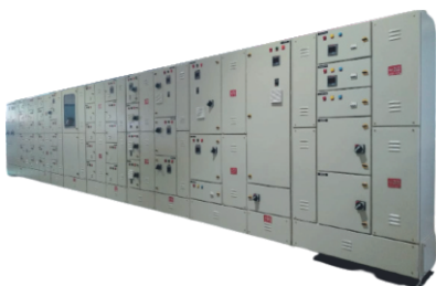
AC Drive Panels
