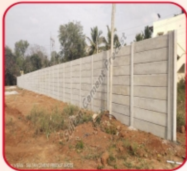
Precast Concrete Compound Wall
