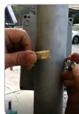
4- Fix the tape around the mast
