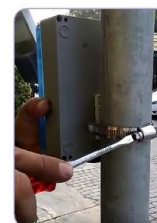
5- Tighten the tape with a screwdriver
