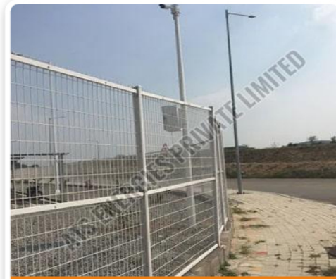
Mild Steel CCTV Camera Pole
