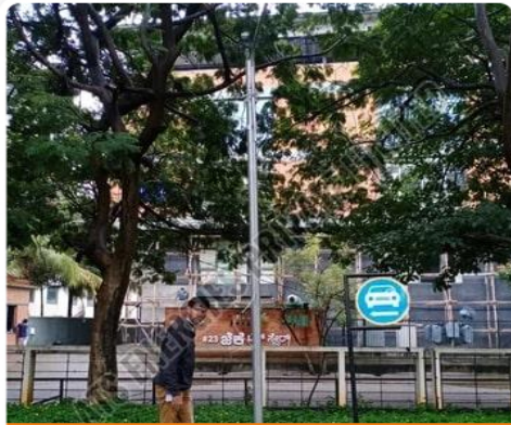
Galvanized Iron CCTV Camera Pole
