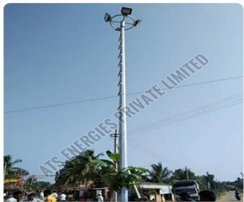
Mild Steel High Mast Pole
