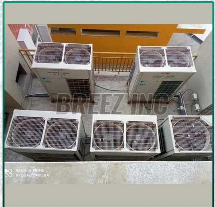
VRV Air Conditioning System
