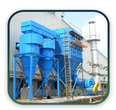
A dust collection system is an industrial air quality control system designed to capture and remove airborne dust and particulate matter generated during various manufacturing and industrial processes to prevent the release of pollutants into the atmosphere.
