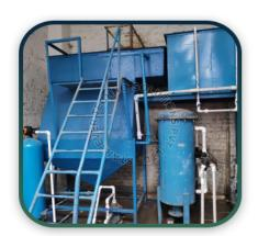
An Effluent Treatment Plant (ETP) is a facility designed to treat and manage industrial wastewater, also known as effluent. The primary goal of an ETP is to remove pollutants and contaminants from industrial wastewater before it is discharged into the environment or municipal sewage systems.
