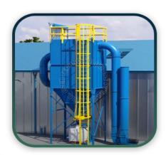
A baghouse filter, also known as a fabric filter or dust collector, is an air pollution control device designed to capture and remove particulate matter (dust) from industrial gas streams. It is a key component of dust collection systems and is widely used in various industries to enhance air quality and comply with environmental regulations.
