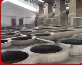
Commercial Jaggery Plant
