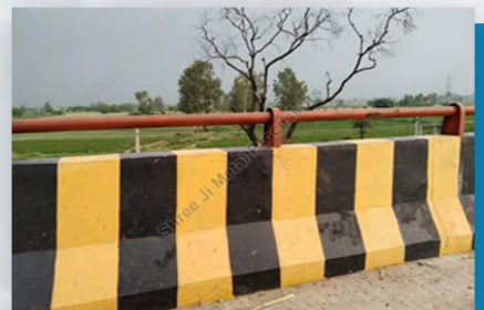
Bar Road Side Steel Railing
