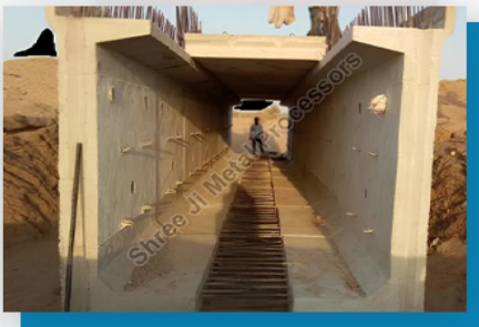
RCC Box Culverts
