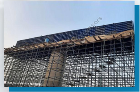
Pier Cap Formwork Shutter
