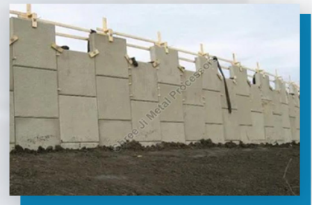
Soil Retaining Wall
