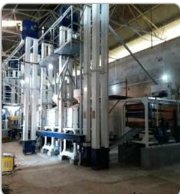
Rice Mill Plant
