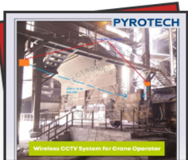
Wireless CCTV System for Crane Operator
