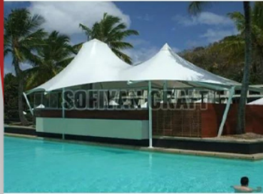
Swimming Pool Tensile Structure
