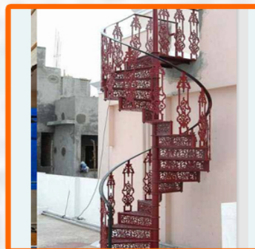
CAST IRON STAIRCASE
