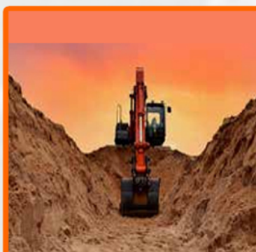
Excavation & Foundation Work
