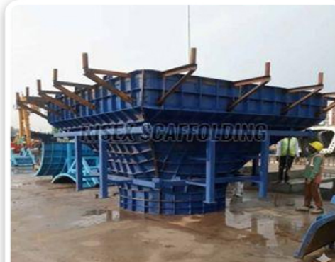
Pier Cap Shutter
