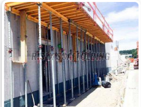
Slab Formwork System
