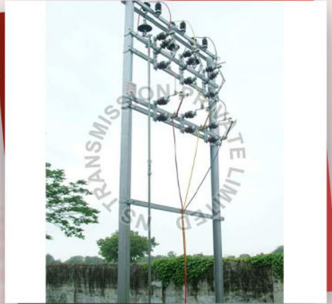
Double Pole Structure
