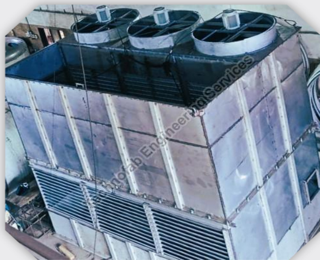
CLOSED LOOP COOLING TOWER
