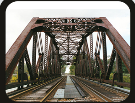
Railway Bridge Fabrication Services
