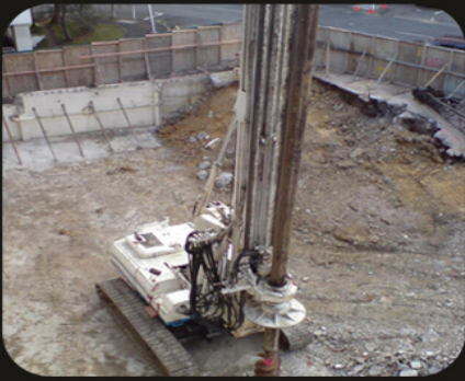
Pile Foundation Services
