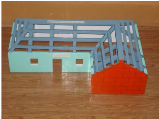
Roof showing Ridge , Hip & Valley
