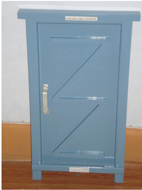
Ledger & Braced Door with Frame
