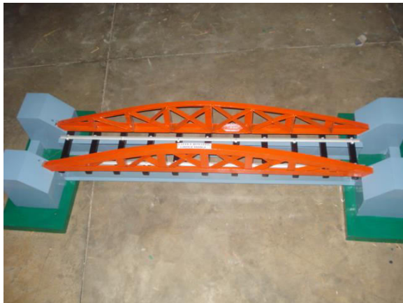
Lattice Bowstring Girder Bridge
