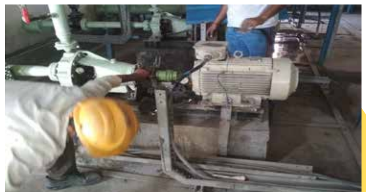
REPAIR AND MAINTENANCE OF ASH HANDLING PUMPS PROJECT AT ANNUPUR, MADHEYA PRADESH
