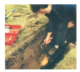
HEAT SHRINKABLE Cable Jointing & Terminating systems have covered all the installation difficulties to make it most easy to use and most effective in gruelling environmental conditions. These are reliable, easy and fast to install and can be relied on for years of trouble free service.
