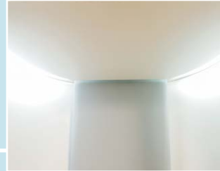
Controllable dimmed ceiling downlighting
