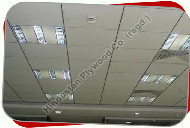
CALCIUM SILICATE BOARD FALSE CEILING
