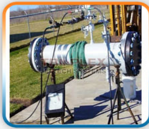
Hydro Testing Service
