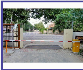
Automatic Boom Barrier Gate
