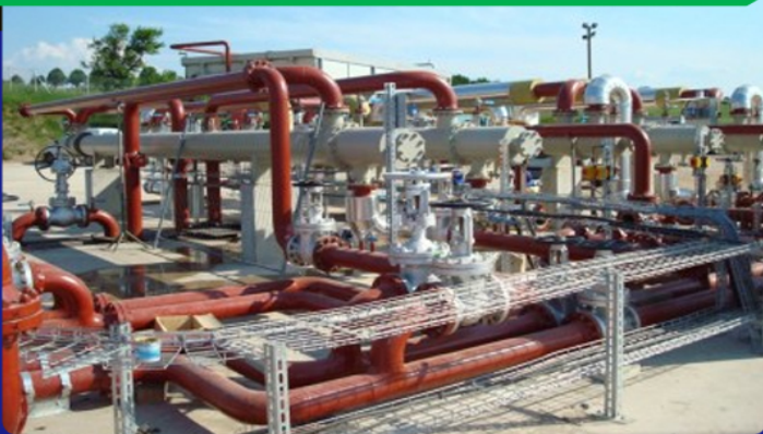
Industrial Plant Electrical Work Services
