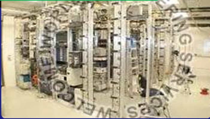
Plant Electrical Work Services
