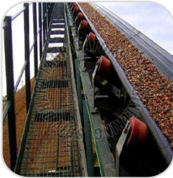
Material Handling Conveyor System
