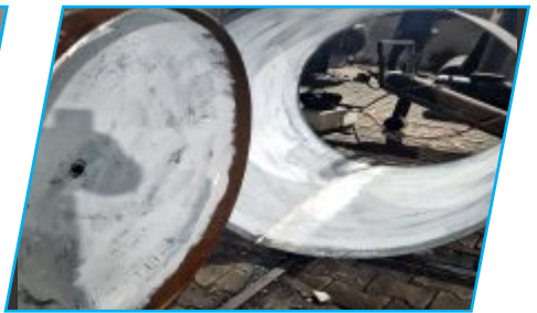
Epoxy Coating Inside Tanks
