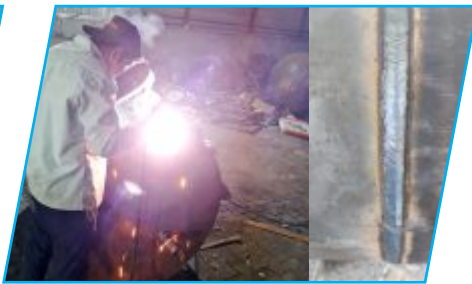
Welding Process by Skilled Operator
