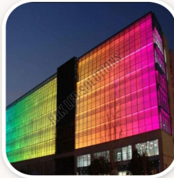
LED Building Facade Lighting
