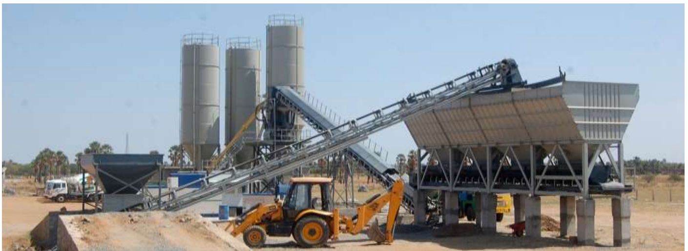
Concrete Batching Plant
