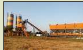
CONCRETE BATCHING PLANT
