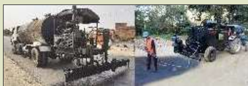
BITUMEN / EMULSION SPRAYER
