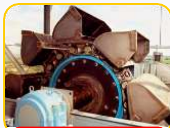
Elevator Bucket & Chain
