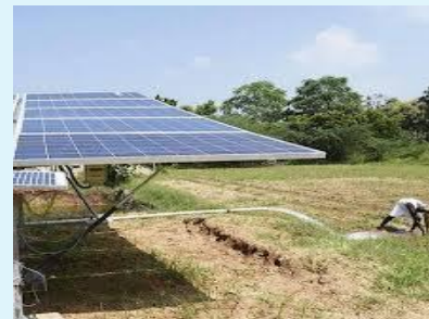
Solar Water Pumping Systems
