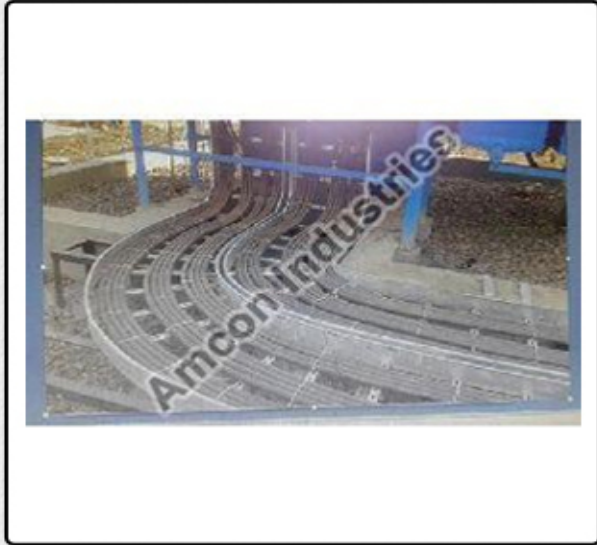
90 Degree Cable Tray Bend
