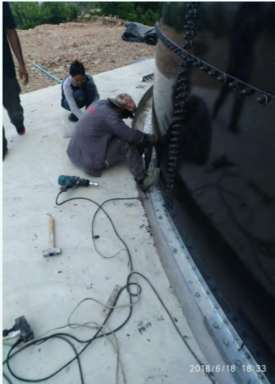
Install the base angles
