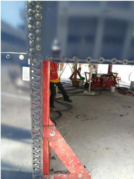
Apply the Sealant
