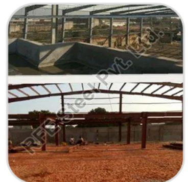
Badminton Court Roofing Shed
