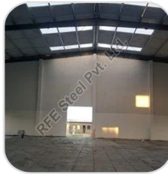
Prefabricated Roofing Shed
