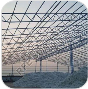
Warehouse Roofing Shed
