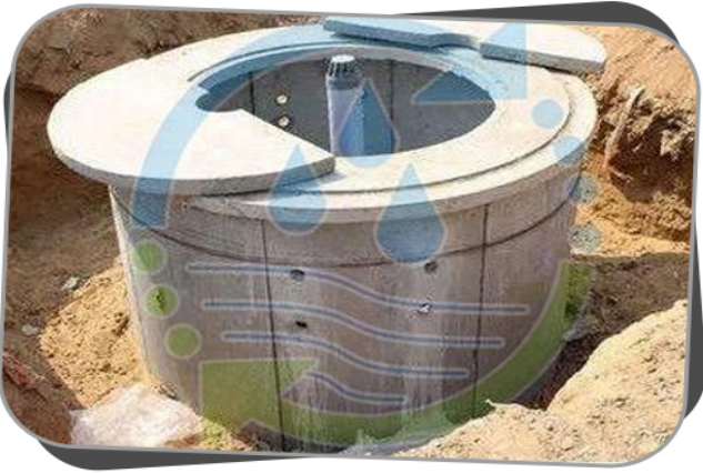
RAINWATER HARVESTING RECHARGE WELL
