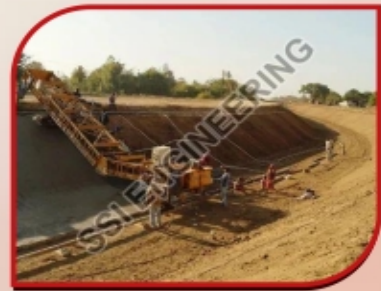
Canal Slope Paver Machine
