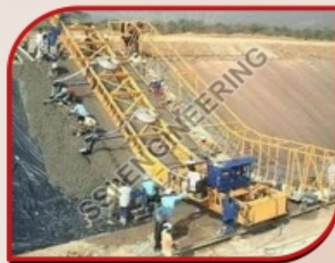
SSI Engineering Canal Paver Machine
