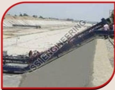
Automatic Concrete Canal Paver Machine
