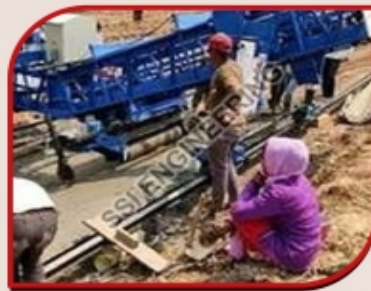
Automatic Concrete Lining Canal Paver Machine
