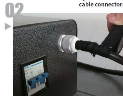
02 Insulation and repair of cables
