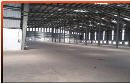
50000 Sq. Ft. Industrial Shed For Rent In Khatraj, Ahmedabad
