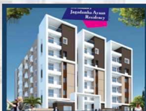
Jagadamba Ayaan Residency Type : Flats & Apartments
