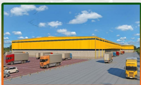
Warehouse In Logistics Parka At Palwal Haryana On BTS Model
