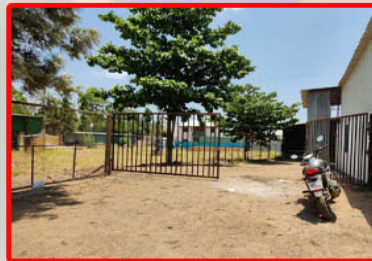
20000 Square Feet Industrial Shade For Rent In Malegaon MIDC, Sinnar, Nashik
